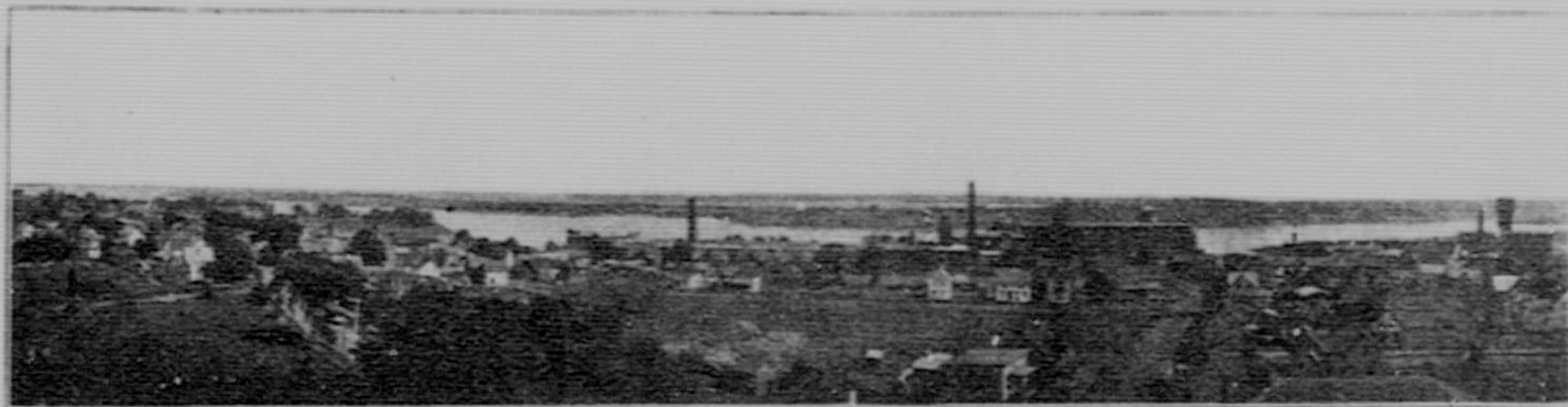
Cornwall East from Tower of Church of the Nativity.
