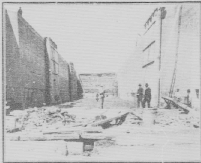
Cornwall Lock 18, unwatered for repairing bottom. The water is shut out by a temporary dam, as seen in the distance.
