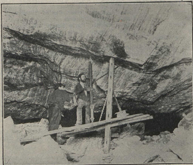
Drilling for Blasting
