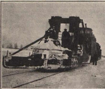
Fig. 2. Spreader with extension nose attached.
