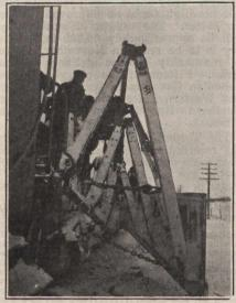
Spreader with wing chained for final widening of 6 ft. 4 in. from rail.
