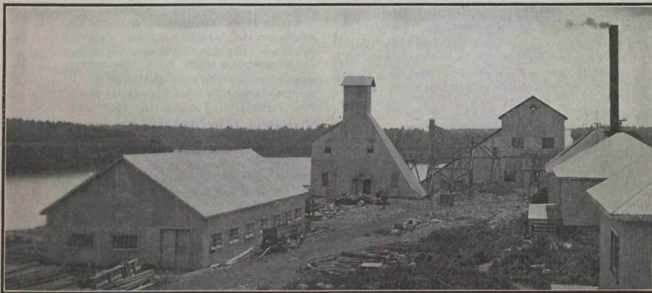
General View of Plant, Swastika Mine, Ont.
