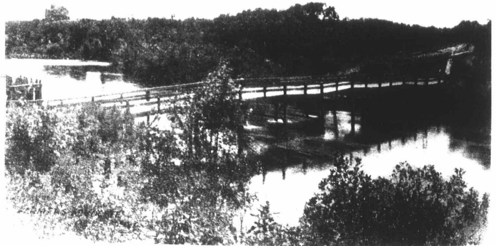
TEMPORARY BRIDGE OVER THE SOURIS RIVER AT SOURIS.
