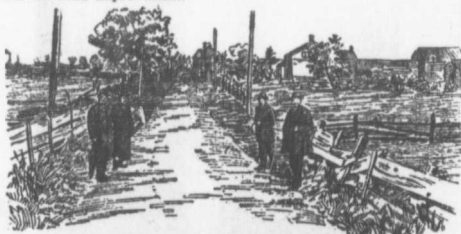
Road near Kempville, Ont., after being operated on by the good roads train.
