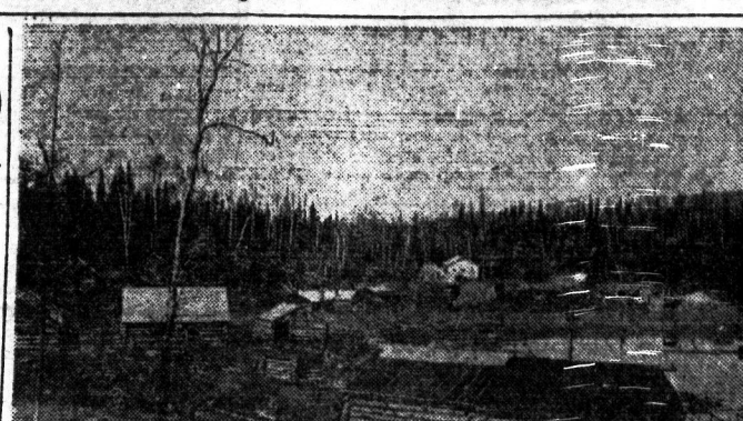
A Section of South Porcupine Destroyed in the Great Fire.
