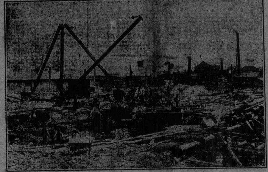
SCENE OF ACTIVITY AT SUGAR REFINERY—SINKING ONE OF THE FORTY-TWO FOOT PIERS FOR THE MELTER HOUSE.
