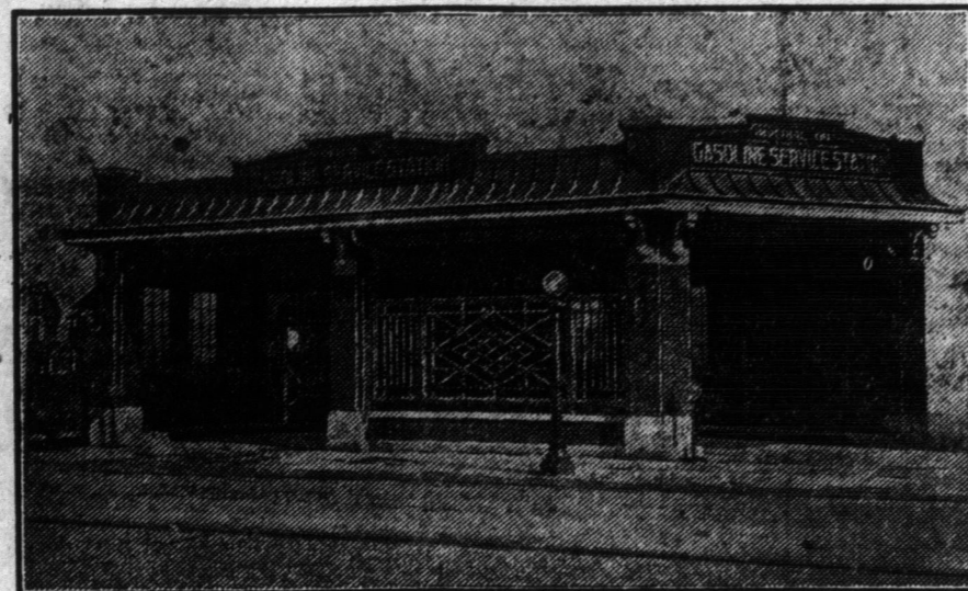
DANFORTH AVENUE IMPERIAL SERVICE STATION Danforth Avenue and Broadview
