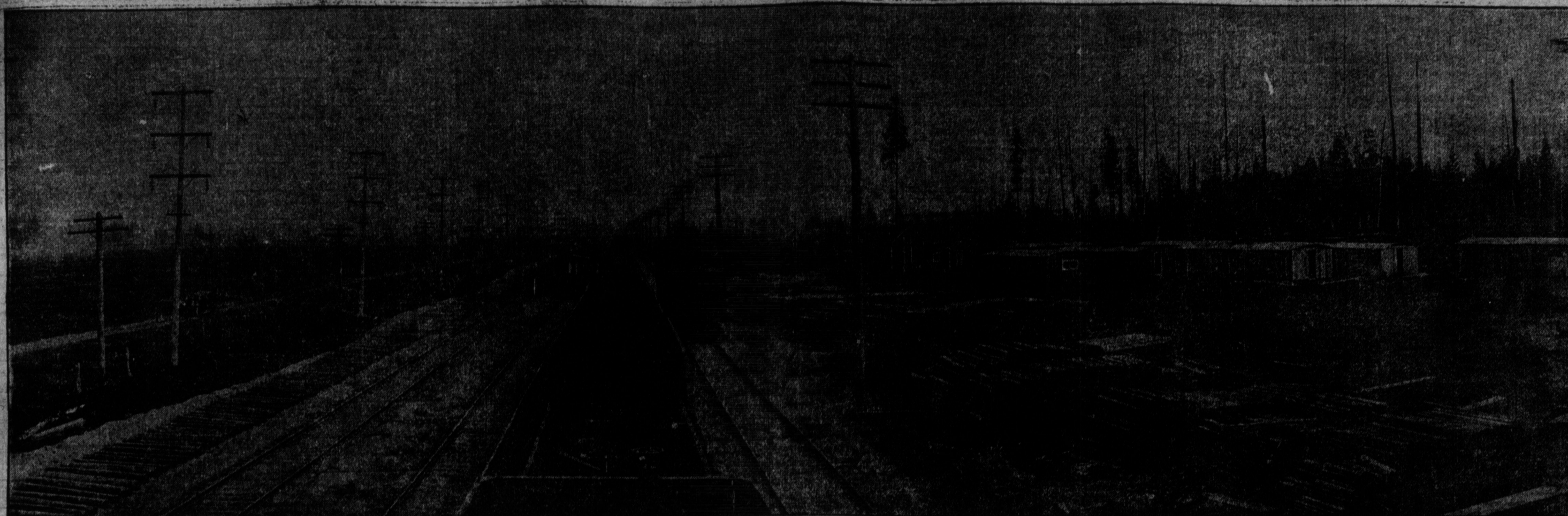
View looking S.E. showing general tracklaying activities along the main line of the C. P. R. at Coquitlam.
