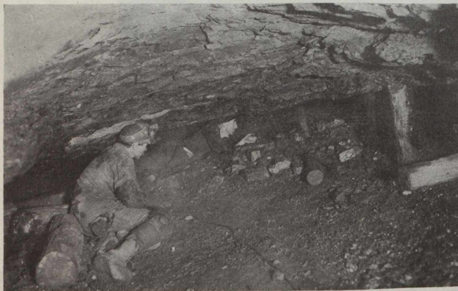
ROCK ROAD OR "CUTTING SIDE" LEADING TO A LONGWALL FACE
