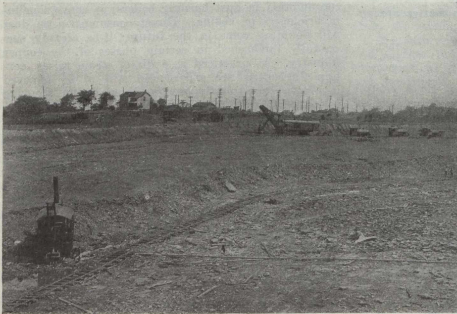
STRIPPING AN ANTHRACITE SEAM
