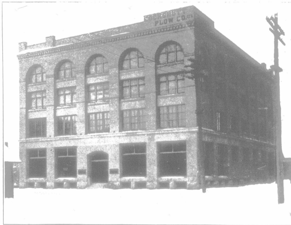
Cockshutt Plow Company Warehouse, Winnipeg.
