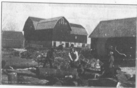
Cutting a Supply of Fuel on a First Prize Ontario Farm*
