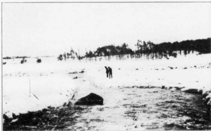
FIG. 31.—Artificial channel blasted through the head-race of a large Power Company to allow of sufficient water-flow.
