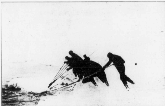
FIG. 32.—Blasting Operation. Men prying off lump which has been cracked off by blast. Frazil underneath.
