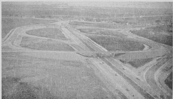
Vancouver-Blaine Freeway showing Westminster Highway Interchange.
