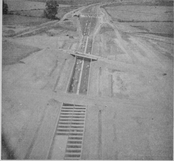
Aerial photograph of Deas Tunnel, showing entrance and exit toll booths.
