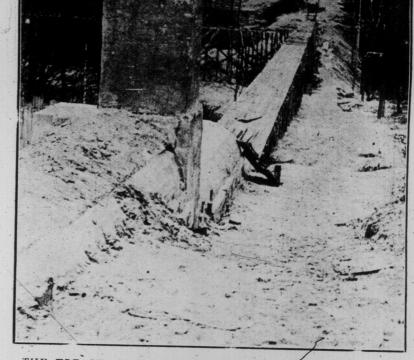
THE TOP OF THIS AERIAL MANHOLE ON THE BLOOR STREET "OVERHEAD" SEWER WILL BE THE NEW STREET LEVEL WHEN THE BIG GULLY AT HIGH PARK IS FILLED IN AND BRIDGED.
