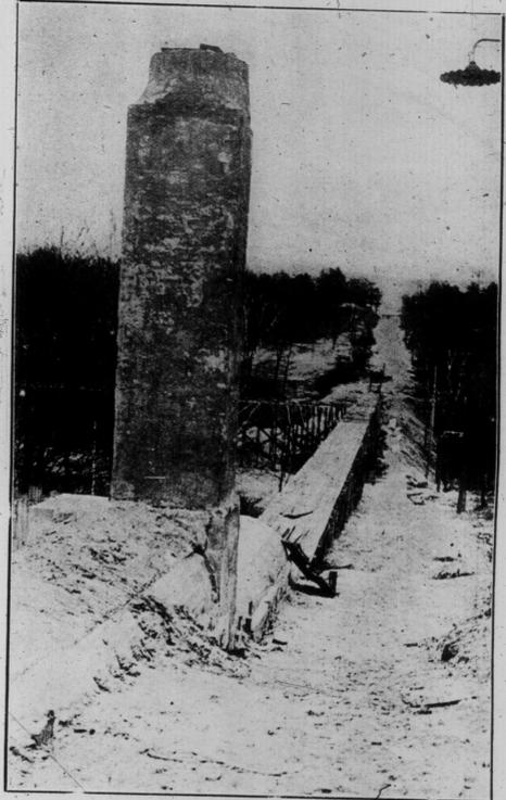
THE TOP OF THIS AERIAL MANHOLE ON THE BLOOR STREET "OVERHEAD" SEWER WILL BE THE NEW STREET LEVEL WHEN THE BIG GULLY AT HIGH PARK IS FILLED IN AND BRIDGED.
