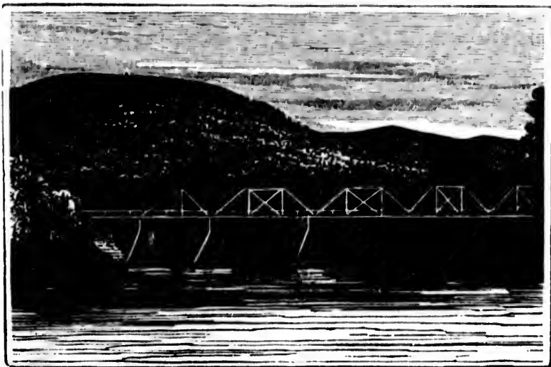
Rumford Bridge, Androsoggin River.
