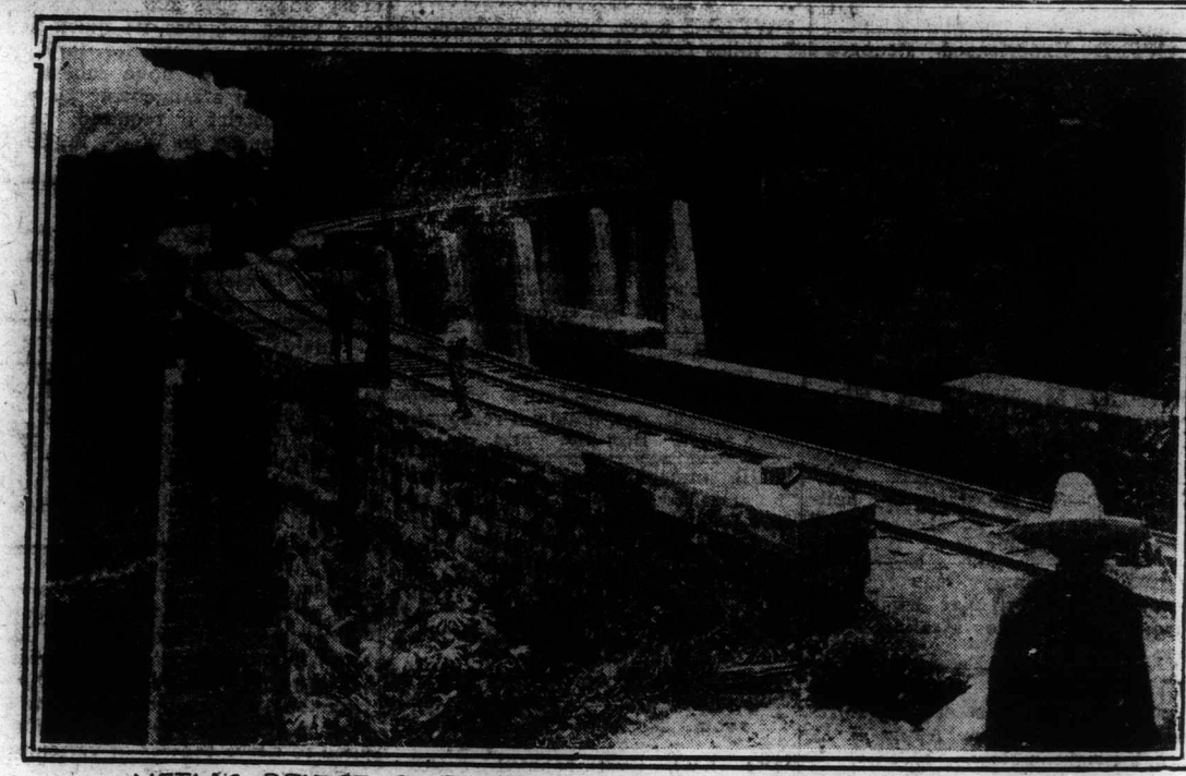
METLAC BRIDGE ON RAILROAD BETWEEN VERA CRUZ AND MEXICO CITY.
