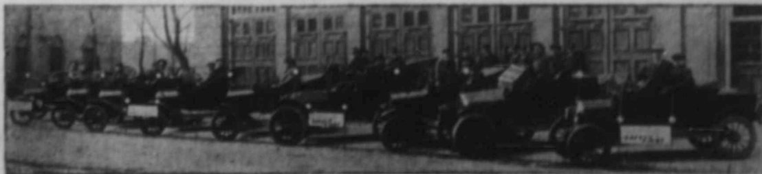
One of Our Installing Divisions
