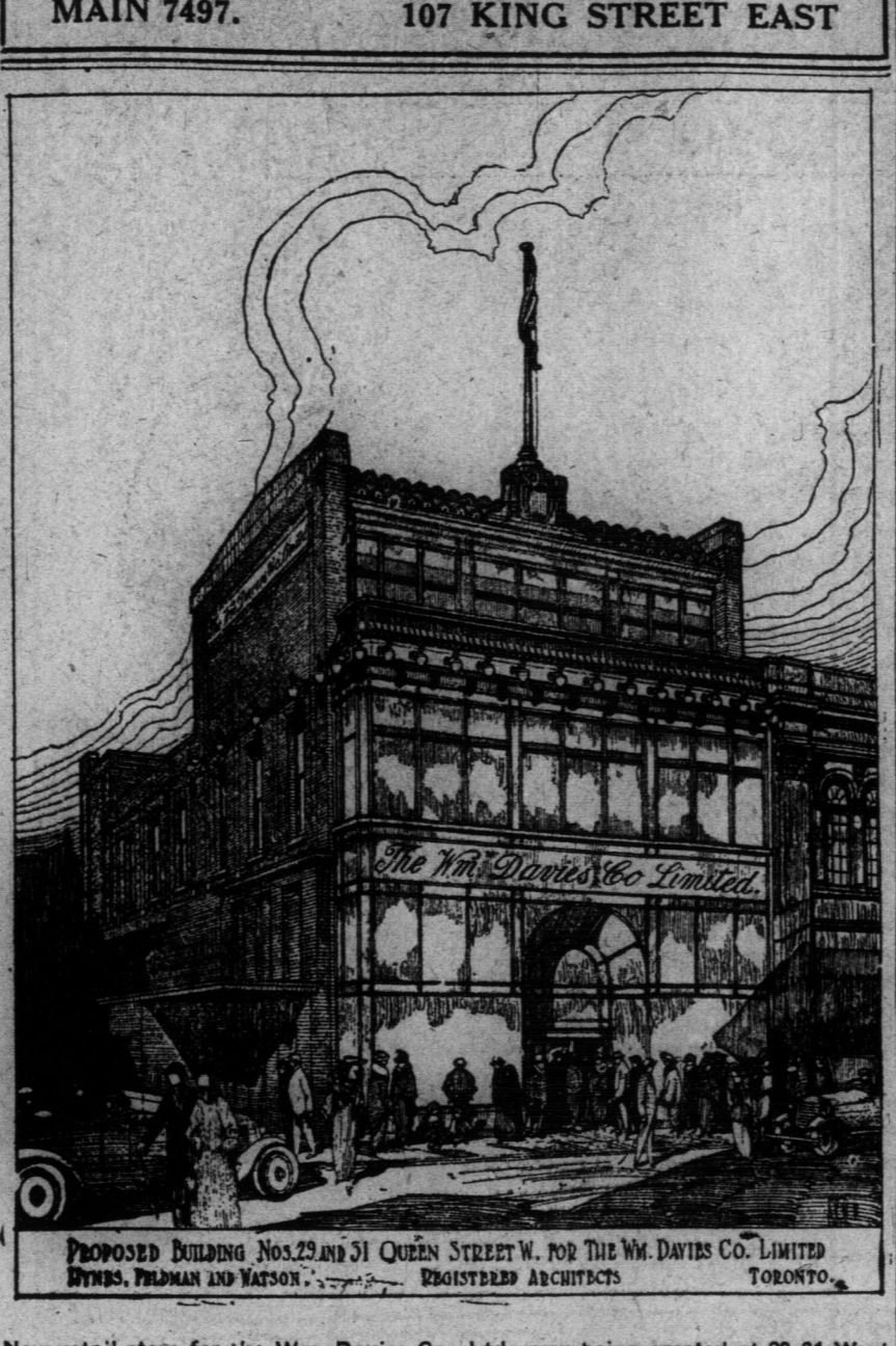
PROPOSED BUILDING NOS. 29 AND 31 QUEEN STREET W. FOR THE WM. DAVIES CO. LIMITED BYRNE, FULMAN AND VANDERSON, REGISTERED ARCHITECTS TORONTO.
