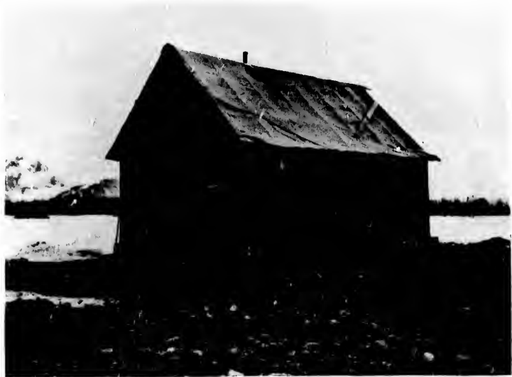
10.—KITCHEN OF HOSPITAL FOR DESTITUTE MINERS AT VALDEZ. MAY 9, 1899.
