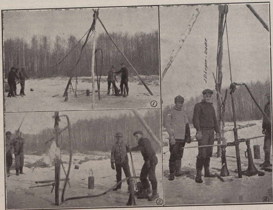
Fig. 1.—General View of Outfit. Fig. 2.—“Drilling.” Fig. 4.—Jacks, used only to raise casing after drive weight has been in operation.
