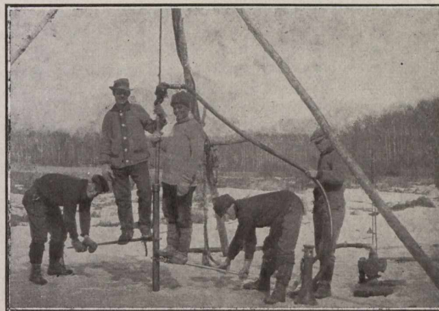
Fig. 3.—Showing Method of Rotating and Sinking the Casing.
