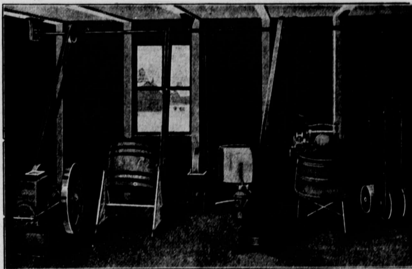
By the installation of a lineshaft in the basement a very great amount of the drudgery of household work can be done away with
