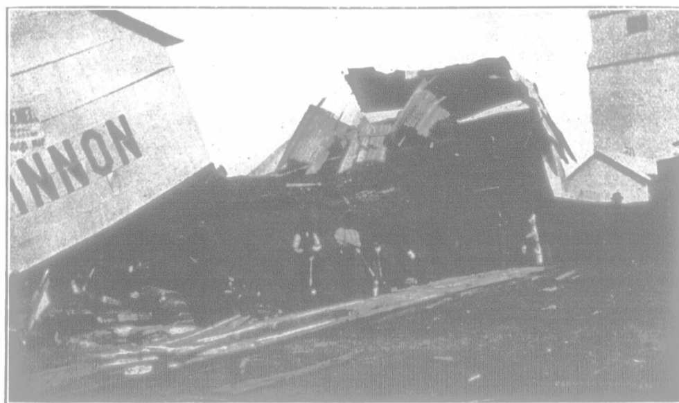
A SLUMP IN WHEAT. The Elevator that Collapsed.
