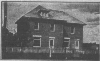
The Electrified Home of G. V. Taylor, Hastings Co., Ont.
