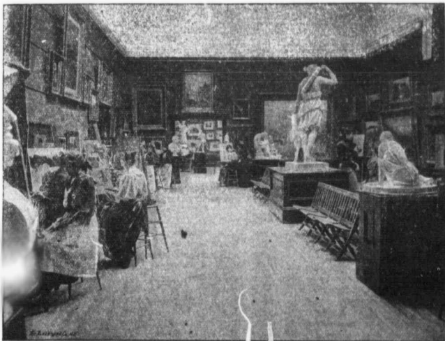
INTERIOR OF ART BUILDING BROCKVILLE.
