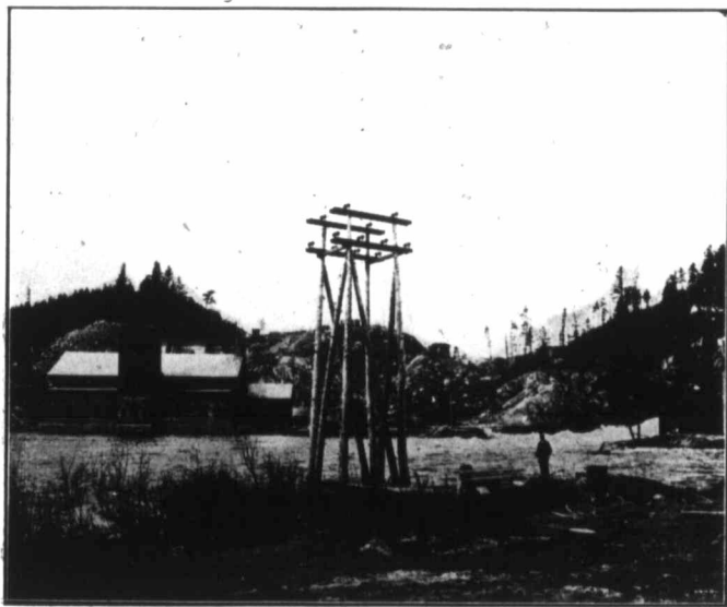
Power Station, High Falls.
