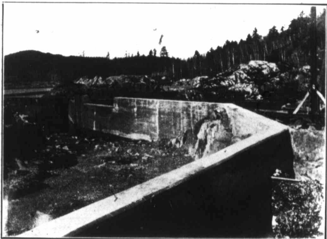
No. 3 Dam and Forebay.
