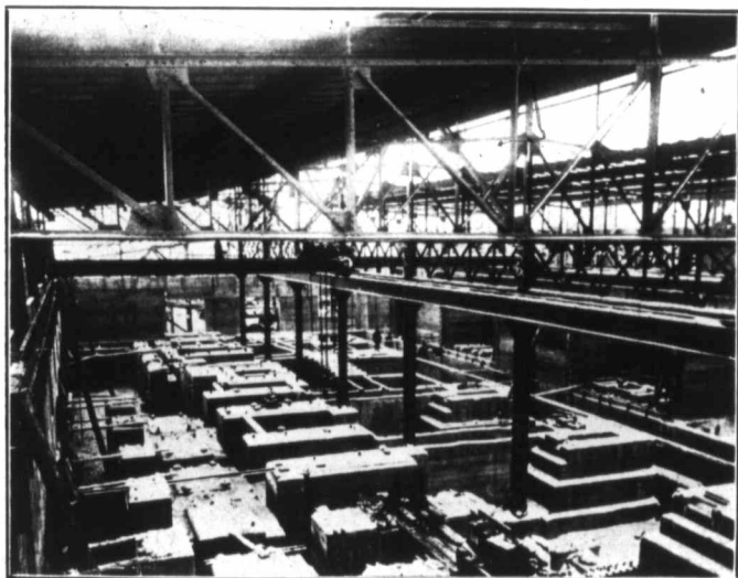
Main Sub-Station, Copper Cliff.
