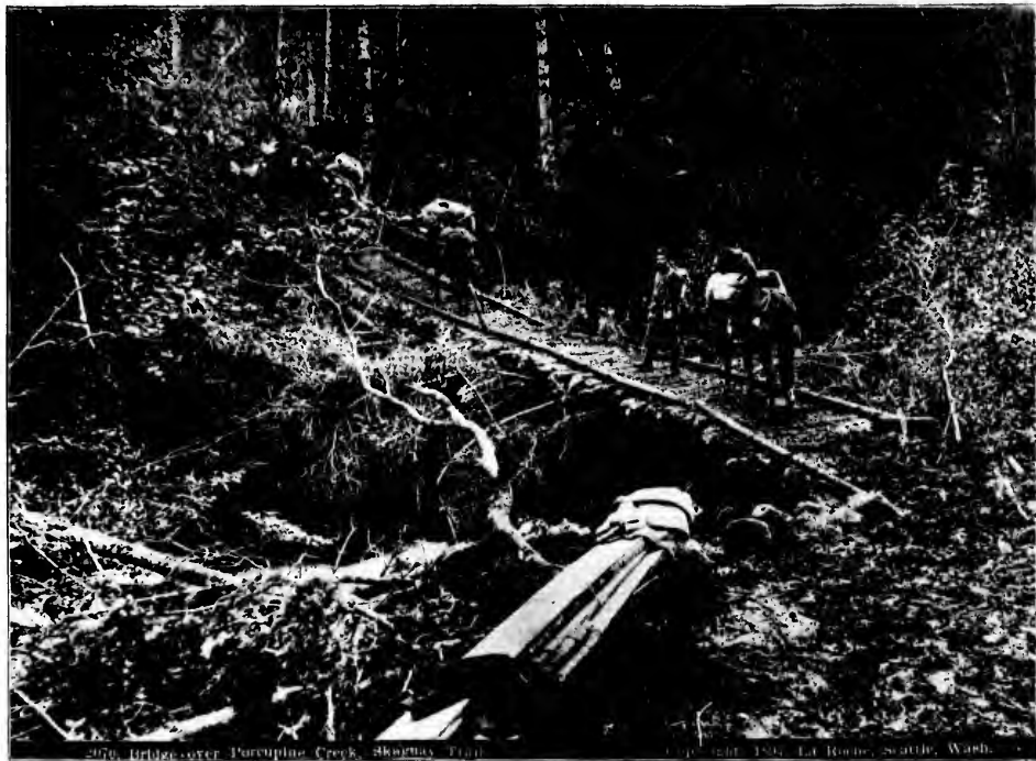
2070. Bridge over Porcupine Creek, Skaguay Trail.
