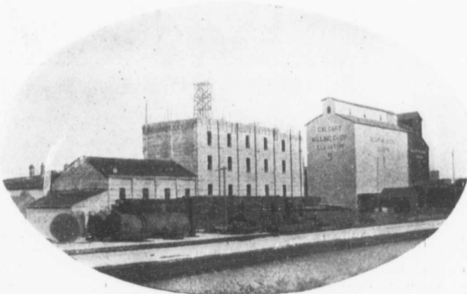
Calgary Milling Co's Elevators and 1,000 bbl. Flour Mill.
