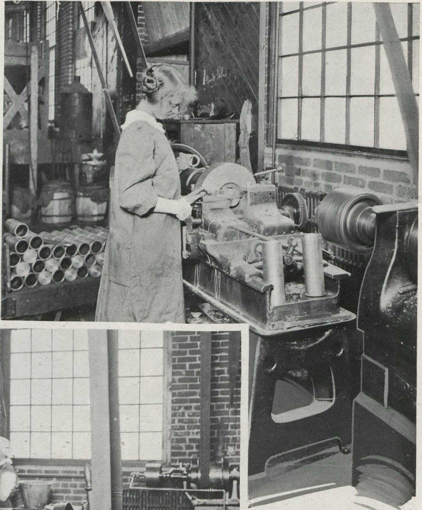
Cutting Off the Base 18-pounder Shrapnel
