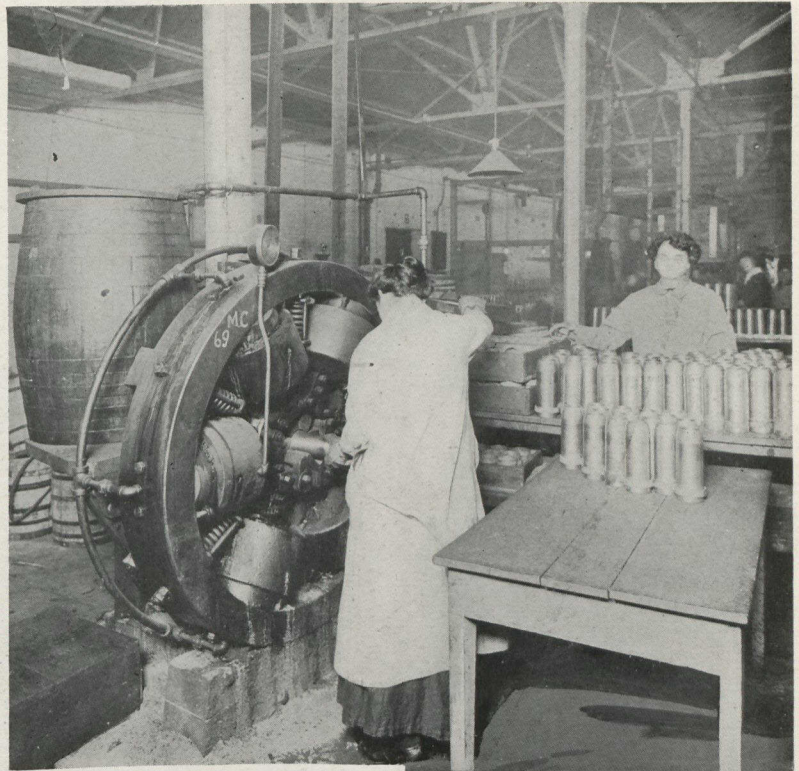
Pressing on the Copper Driving Band with Hydraulic Press
