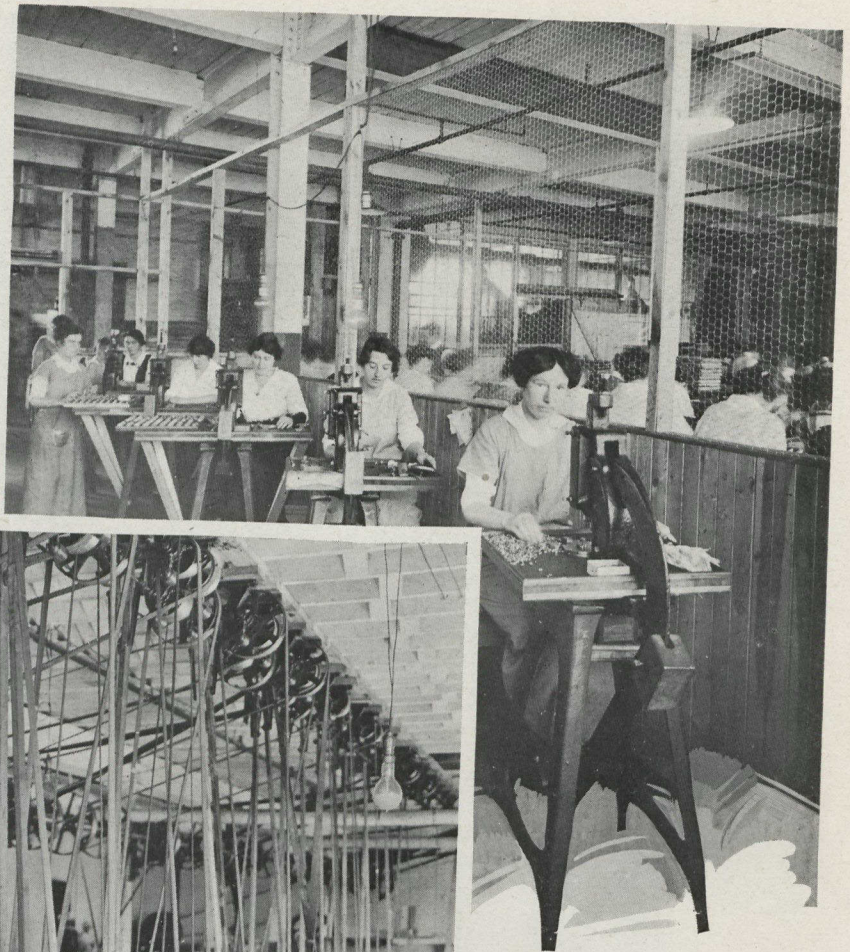
Foot Presses. Pressing Needles in Needle Plug.
