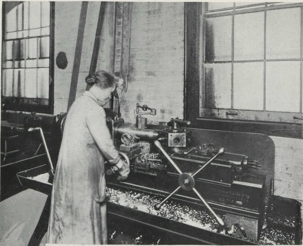
Turning Copper Driving Band
