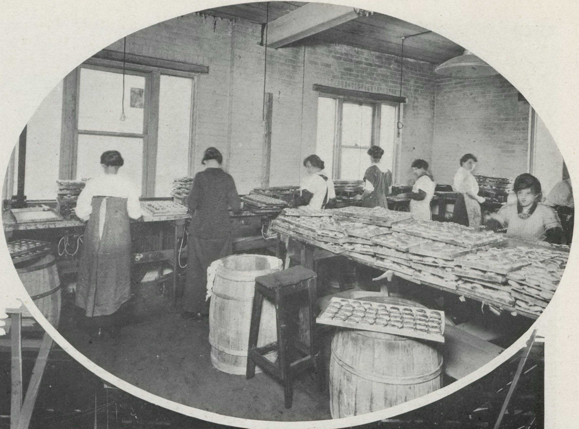
Soldering Powder Cans for 18 Pounder Shrapnel Shells.
