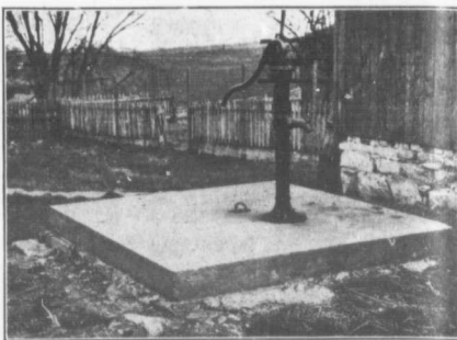
A Home-made Well Platform that is Cheap and Durable
