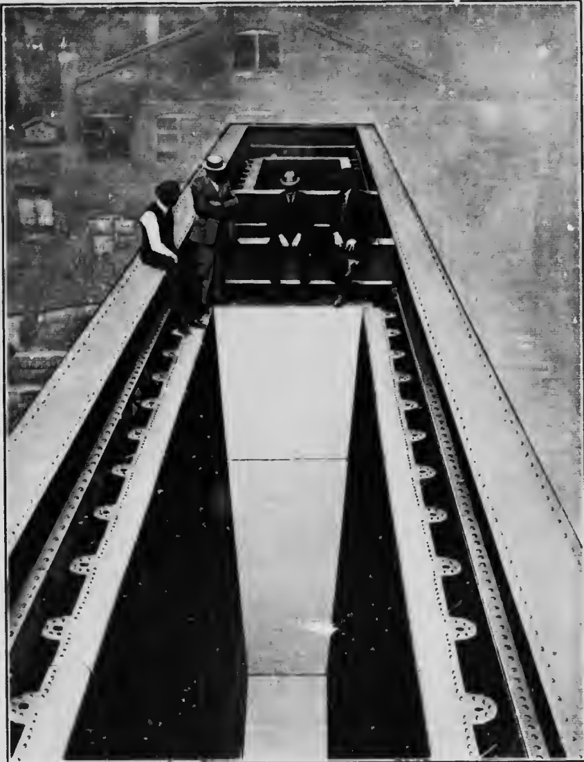
Interior of a blast furnace, Anyox plant, Granby Consolidated Mining and Smelting Co., Anyox, B.C.
