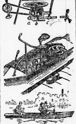
motion of the pedals, a backward or forward movement or even a complete stope page, if the shaft be given an intermediate position. As for the steering, that is affeeted through a bar, analogous to that of bicycles, which controls the rudder.
