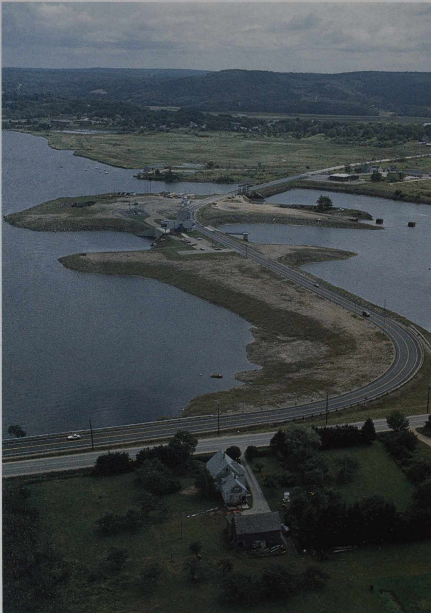
Tidal power generating station at Annapolis Royal
