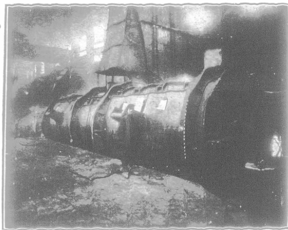
Basic Converter Plant. Latest improvements in Smelting, Copper Cliff
