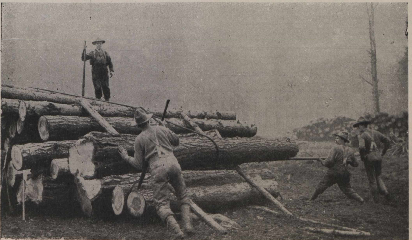
ROLLING A LOG TO THE TOP OF THE SKIDWAY.
