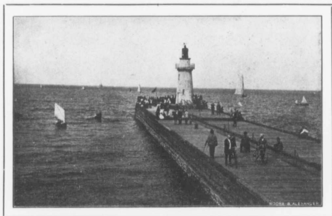
THE PIERS, HAMILTON BEACH
