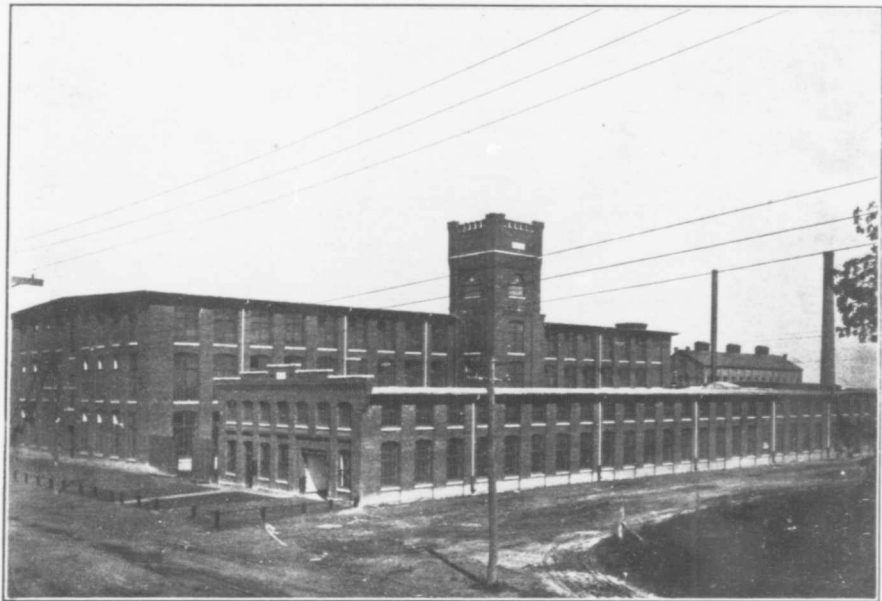
PLANT OF THE IMPERIAL COTTON COMPANY, LIMITED, HAMILTON CANADA
