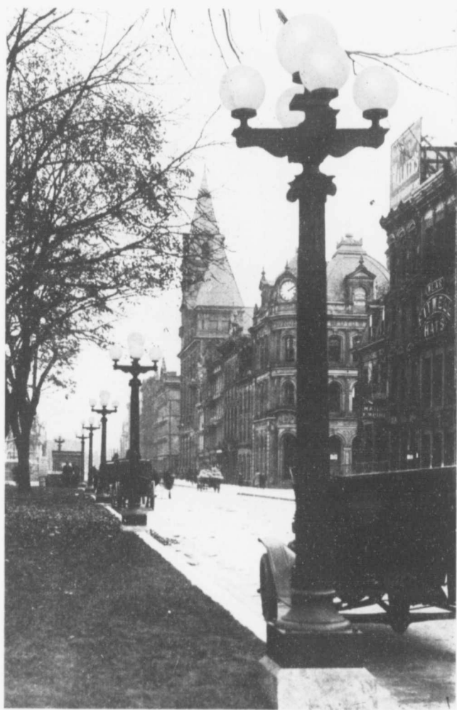
MODERN STREET LIGHTING
