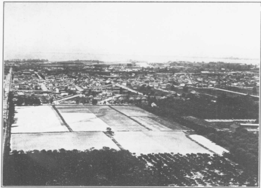
A "NEW HAMILTON"—THE CITY EAST OF TROLLEY STREET
