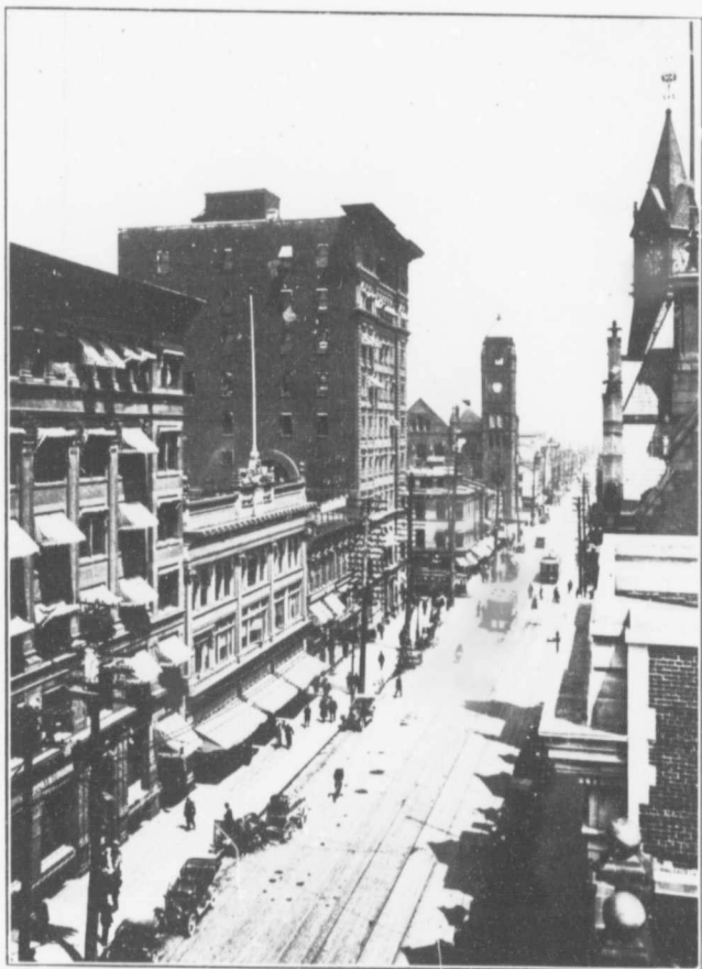
JAMES STREET SOUTH, WEST SIDE.
