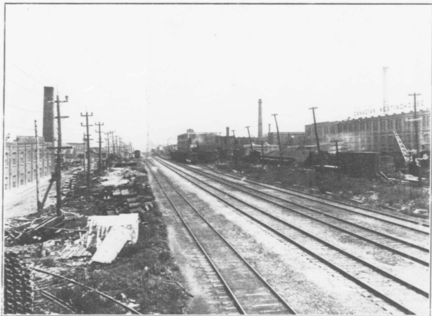
THE GRAND TRUNK DOUBLE TRACK—HAMILTON TO CHICAGO— RUNNING THROUGH THE FACTORY AREA.
