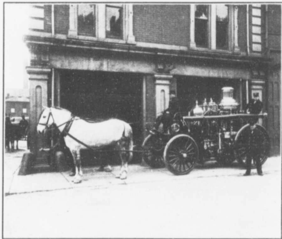
ONE OF THE STEAM FIRE ENGINES
