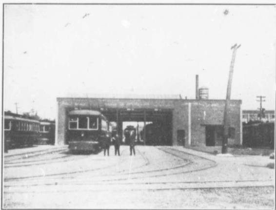
INSPECTION BARN AND STORAGE YARD Hamilton Street Railway Company
