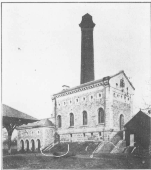
PUMPING HOUSE AT THE BEACH
