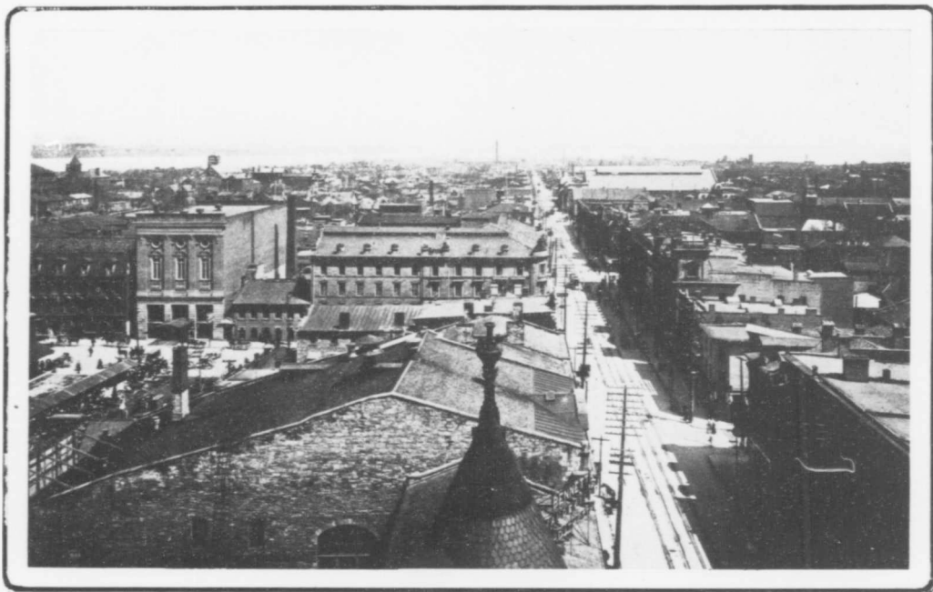
VIEW FROM CITY HALL, LOOKING NORTH
