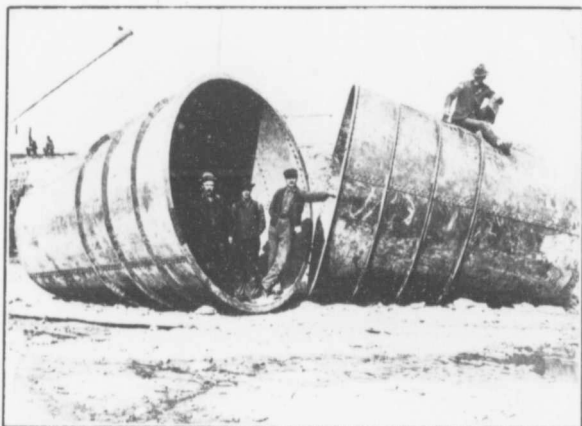
THE HUGE BELLMOUTH INTAKES AT DECEW.
