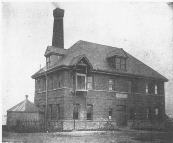
INTERCEPTION WORKS, FERGUSON AVENUE
