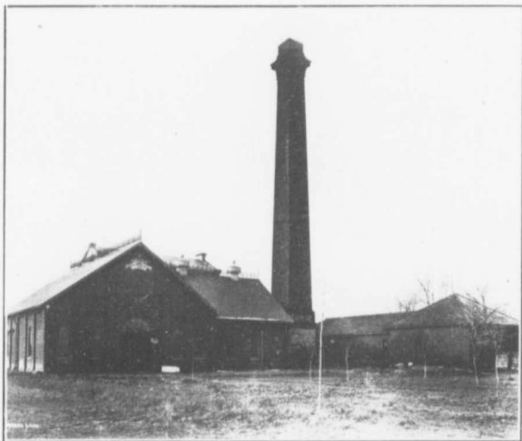
PUMP HOUSE AT THE BEACH
