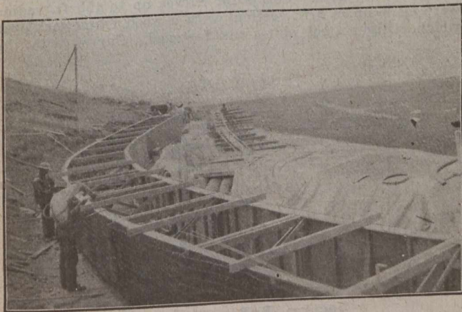
FIG. 1—CONSTRUCTING THE FORMS
