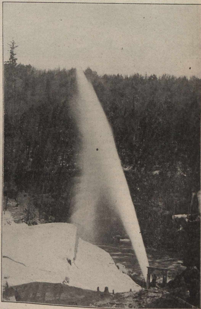
"Blow off," Victoria Mine, on Ontonagon River. The Victoria is one of the pioneers to use hydraulic compressed air. The photo shows a column of water and air escaping from twelve inch pipe, shooting over one hundred feet above the opening.
