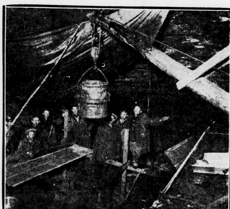
The mouth of the shaft is shown which was dug at Sand Cave, where men worked night and day in an effort to rescue Floyd Collins, imprisoned Kentucky cave explorer
