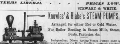
Independent Direct Acting Steam Pumps have a special advantage in Boiler Feeding, inasmuch as speed on be adjusted automatically, or otherwise, to run continuously and maintain water at uniform height. These Pumps can safely be run at speed which makes them an efficient Fire Pump. WISDOM & FISH.
