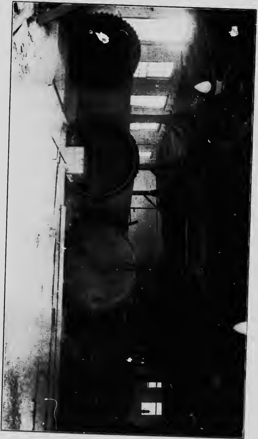
Interior view of the immense cylinders or COOKING OVENS. Cars with 1000 fresh bricks are pushed within them and, after 10 hours under high steam pressure, the bricks are removed fully cured and ready to lay in a structure.
