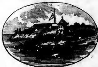
FORT HENRY — MARTELLO TOWER CEDAR ISLAND.
