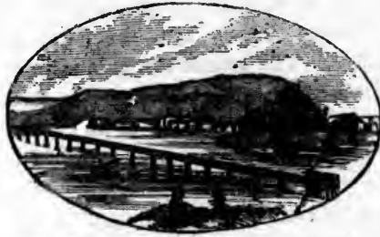
MONTREAL AND VICTORIA BRIDGE.
