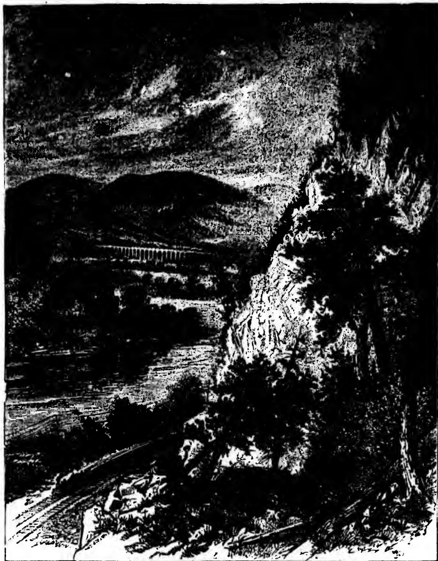
THE STARUCCA VIADUCT.
