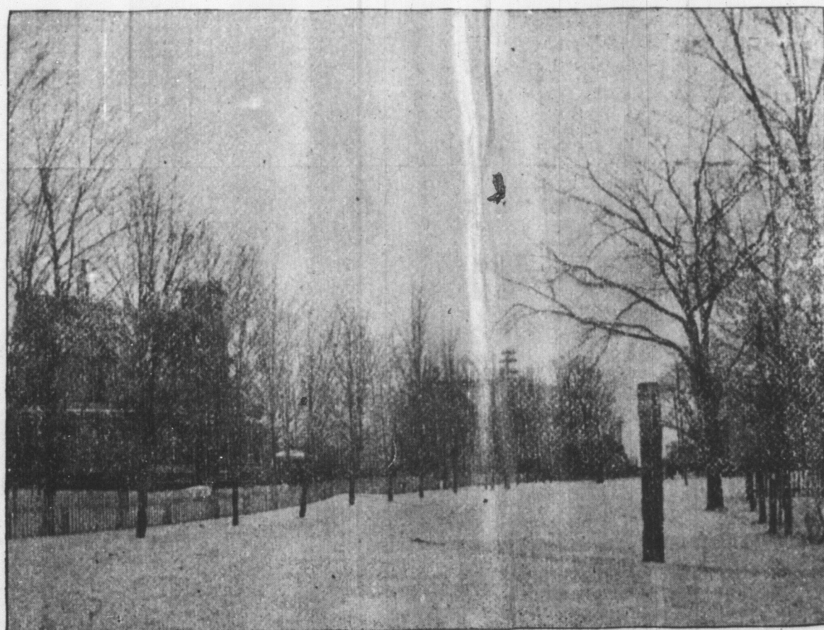
A VIEW OF MAIN STREET, MIDDLETON, NEAR THE CORNER.
