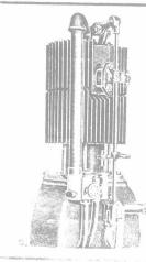
The Air-Cooled engines have failed because the small radiating surrace will not keep them cool.
