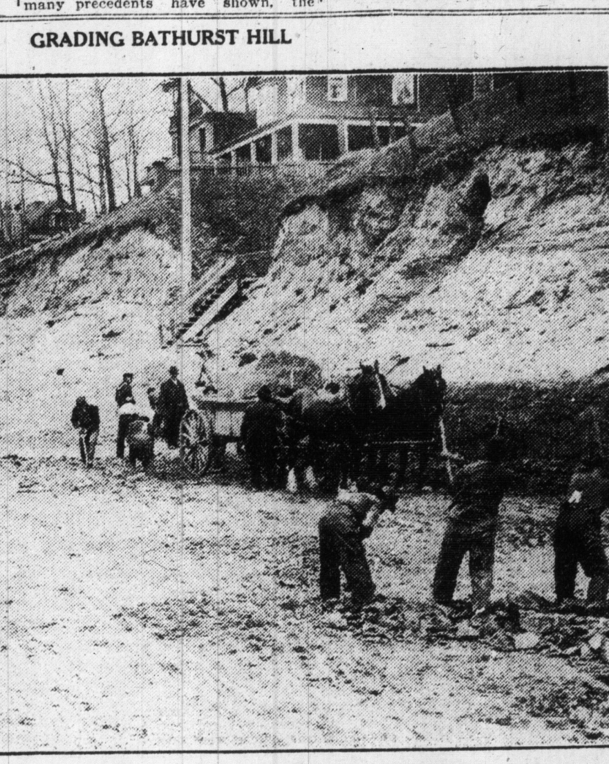
Good progress is being made on the Bathurst hill grading. This photograph shows the depth to which the cutting already has gone.
