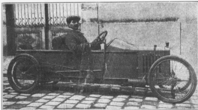
Fig. 287.—The Super, a French Cyclecar Patterned After the Popular Bedelia Model Except That Driver Occupies Front Seat.
